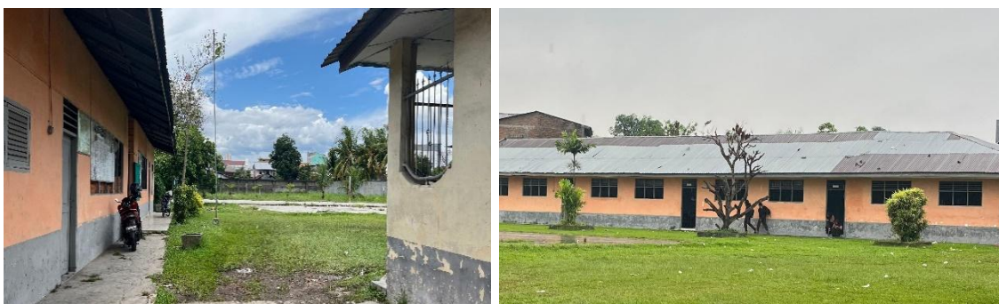
Gambar 1. 2 The atmosphere of Al-Washliyah Middle School in Lalang Village
