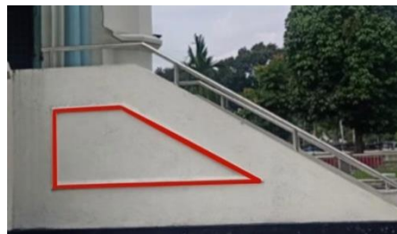
Figure 12. Al-Mashun Great Mosque's Stairs
