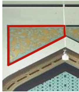
Figure 11. The Ornaments on The Ventilation of The Nazirite Doors
